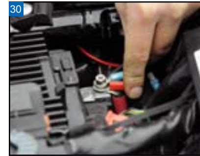
30 Add the power wire from the stabilizer and the Light Wizard harness.
